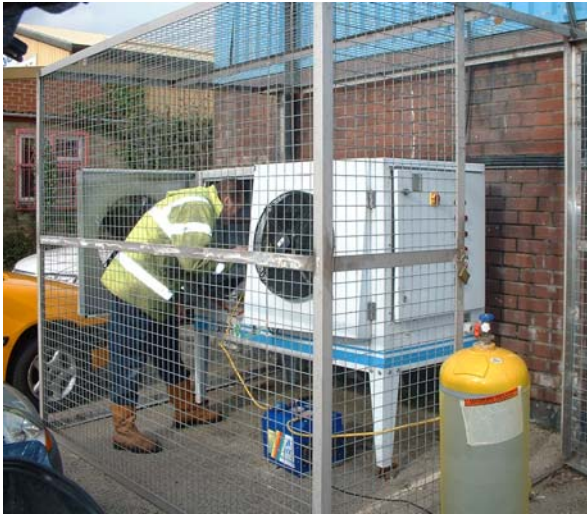
Engineer recovering R404A prior to charging with ISCEON® MO79
